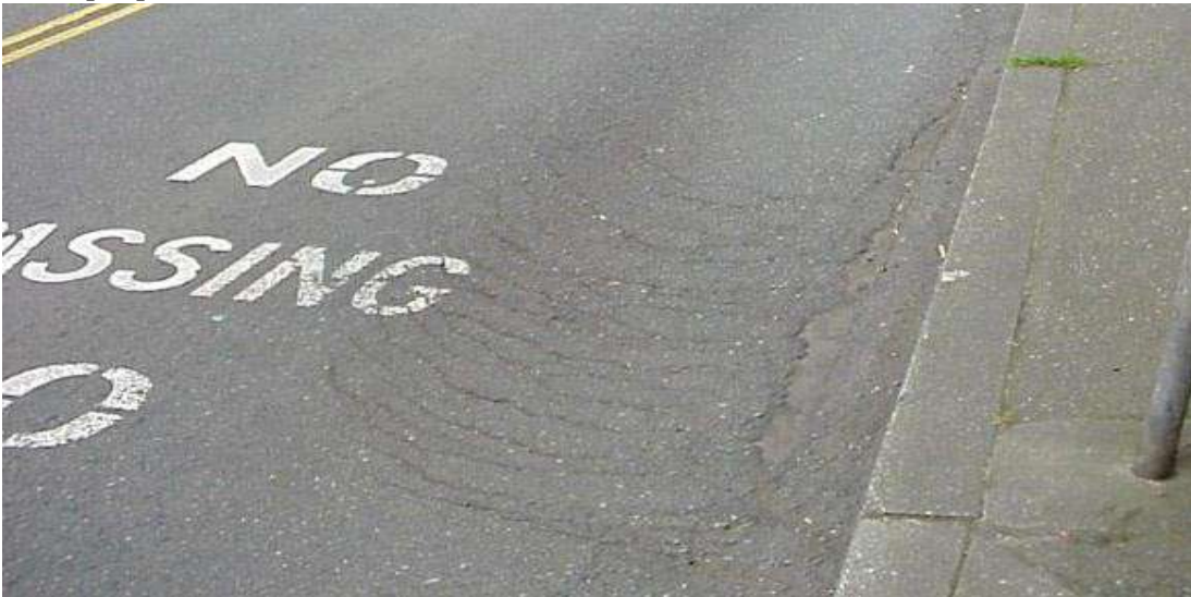
Fig. Slippage Cracks
