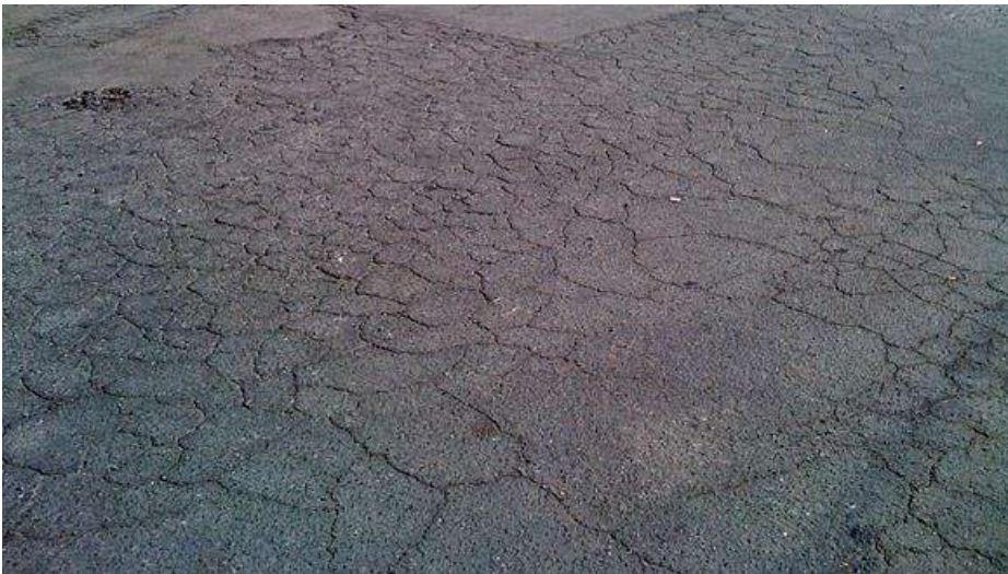
Fig. Alligator Cracking
