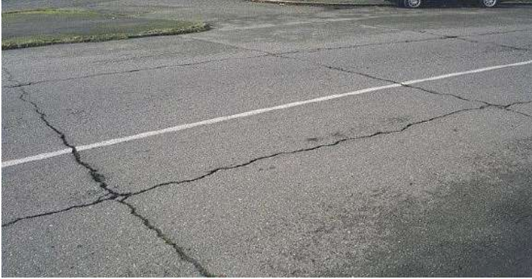
Fig. Joint Reflection Cracks
