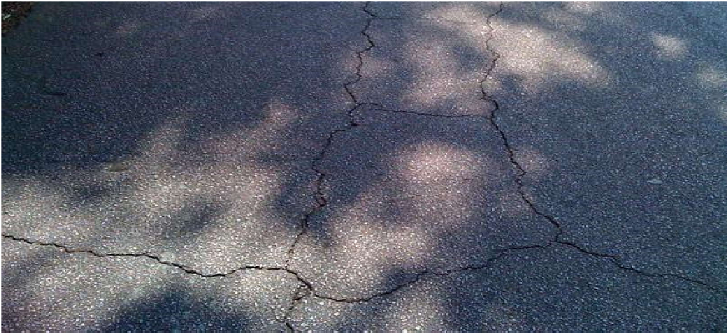
Fig. Block Cracking
