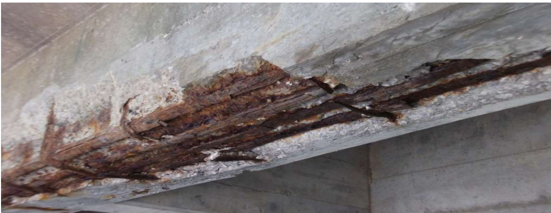
Fig. 1. Corrosion of reinforcing steel is the most common cause of concrete deterioration.
